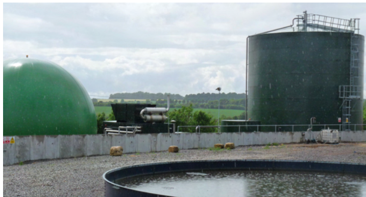
A farm-scale AD plant near Cirencester
